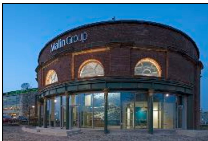
© Paul Zane: Comprehensive repair to enable the reuse of the South Rotunda, GCHT grant of £172,823 towards project costs of £430,592 (Top image: as vacant, bottom image: in use)
