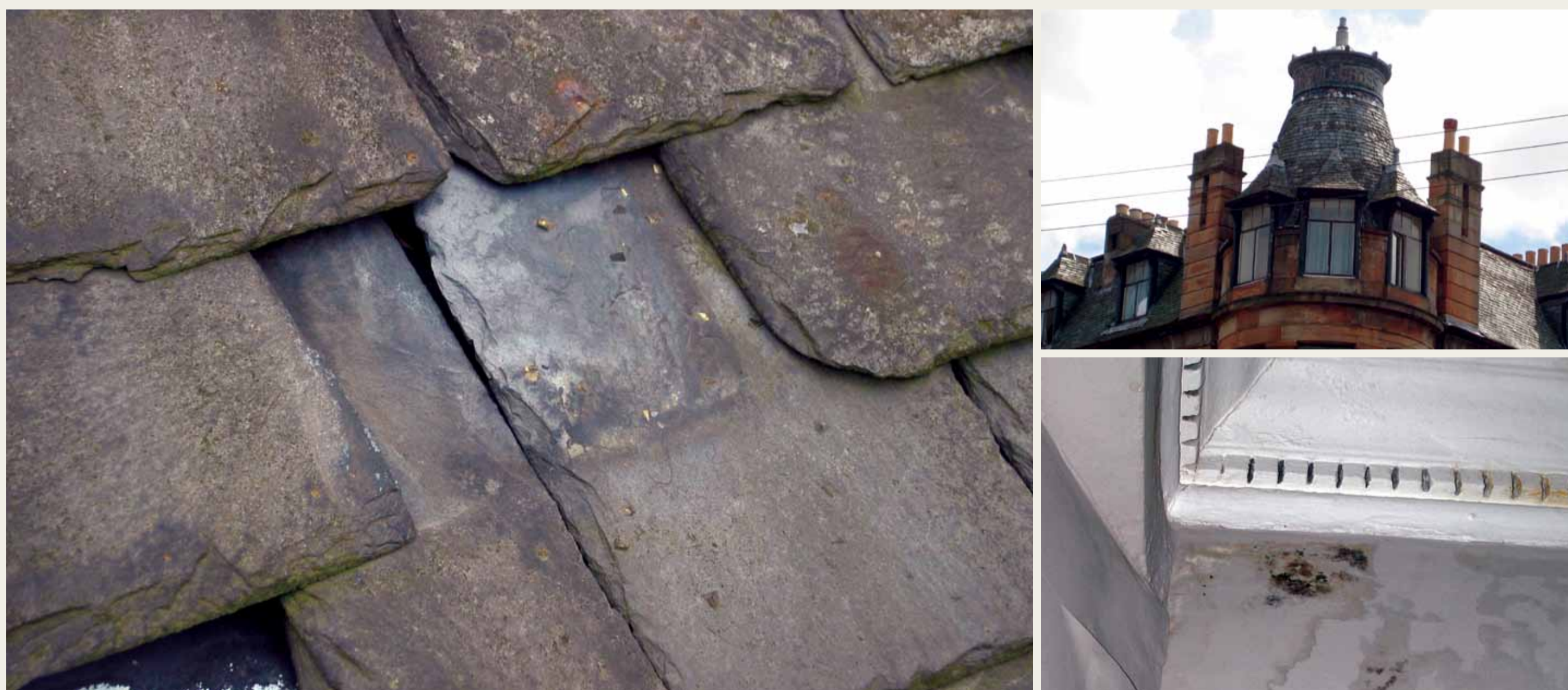
A suitable professional should inspect the roof once a year and replace any missing slates. Victorian slaters were able to create distinctive, flamboyant finishes. Damp on inside walls is often an indication of problems on the roof.
